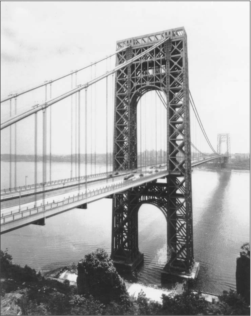
The bridge shortly after it was inaugurated. Note that only the Upper Level is in place. The New Jersey tower, standing on its two river platforms, is in the foreground. Courtesy of Special Collections and University Archives, Rutgers University Libraries.
