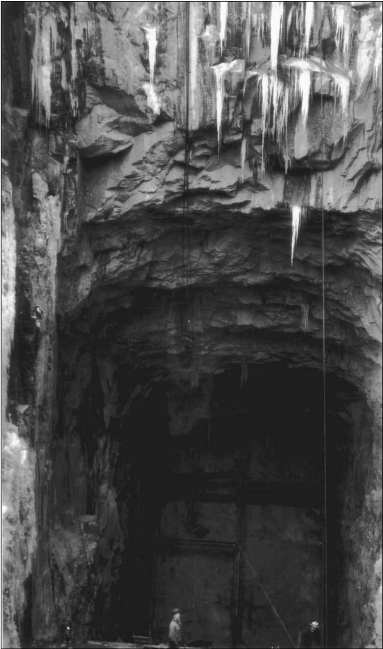
Inside the cavern carved out of the Palisades for the New Jersey anchorage. Courtesy of the Port Authority.
