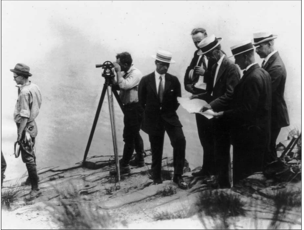
Atop the Palisades with the first surveying work under way. Bridge designer and builder Othmar Ammann is third from the left. Several publications improperly identify Ammann as the man holding the plans, third from the right. This is William Drinker, Port Authority chief engineer. Courtesy of the Local History Department, The Morristown and Morris Township Public Library.
