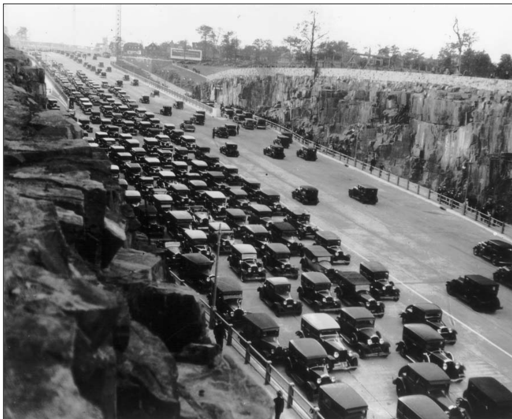
October 25, 1931. Opening Day at the bridge, with cars from New Jersey lined up to pay their fifty-cent toll. Note the rock walls of the Palisades through which the roadway had to be cut. Courtesy of the Local History Department, The Morristown and Morris Township Public Library.
