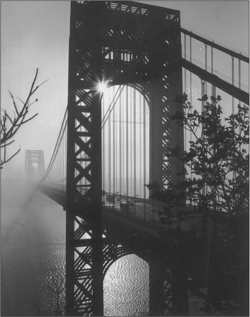
The bridge in fog in 1962, the Lower Level now in place. Courtesy of the Port Authority.
