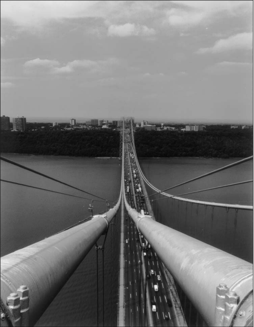
Looking down barrel cables. Courtesy of Dave Frieder.
