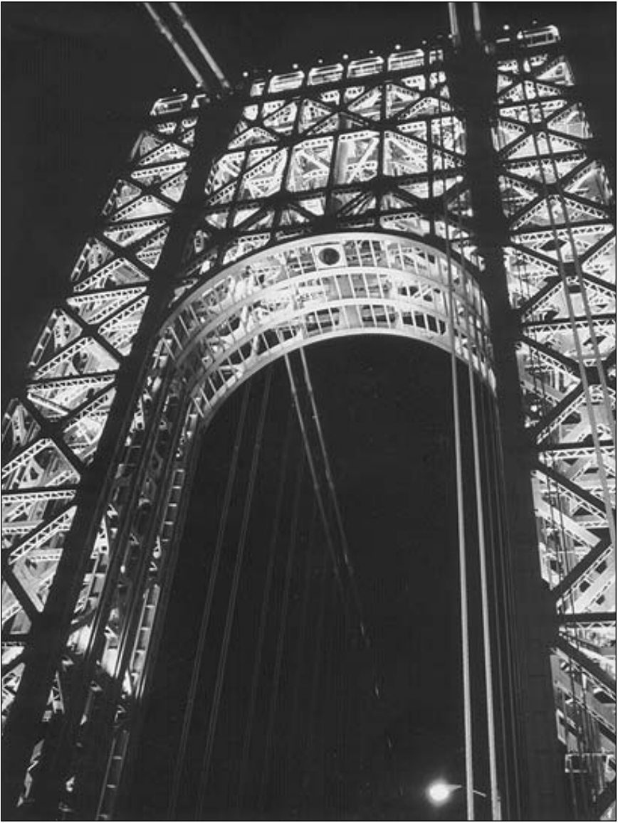
The New Jersey tower after the placement of interior lighting in the year 2000. At the center of the arch underside is the opening of the tube in which the giant sixty-by-ninety-foot flag is stored and from which it is deployed. Courtesy of Dave Frieder.
