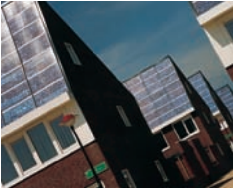
Urban design in the Nieuwland neighbourhood of Amersfoort, Holland, is centred on optimising solar potential
