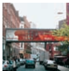
A footbridge links to the adjacent multi-storey car park
