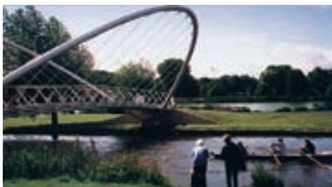
Ouse Bridge, Bedford (Architect: Chris Wilkinson)
