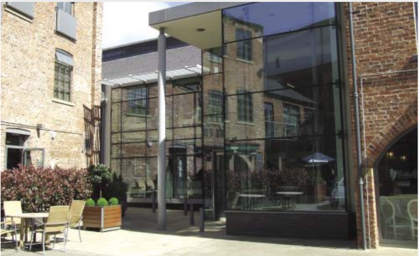
Igloo Regeneration invested in design to attract independent, design-led, creative business occupiers at the Round Foundry, Holbeck Urban Village.
