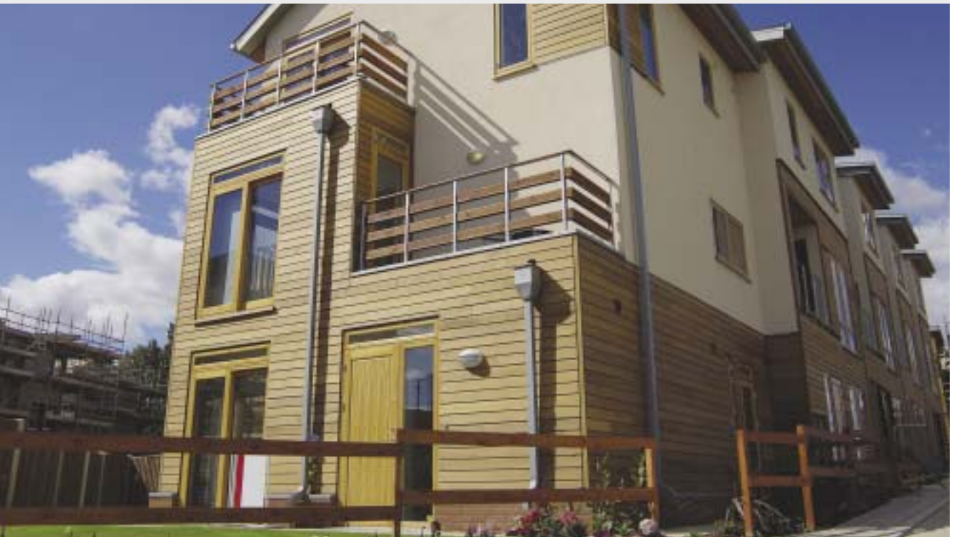
The Summit House at Allerton Bywater was one of the first projects to be built to English Partnerships' Quality Standards.
