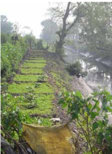
The banks of canals are being upgraded.
