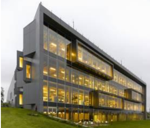
Fig. 3a – Large glazed areas on North face to allow diffused light for office spaces. Source : World Architecture News.com
