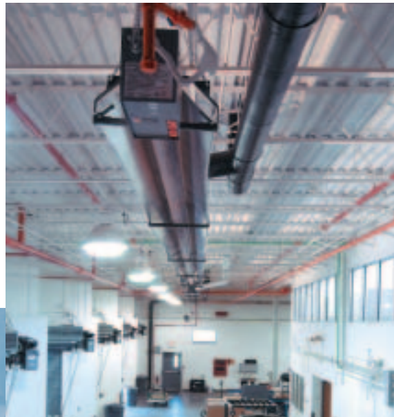
Consider gas-fired radiant heating systems for areas with high ceilings, spot heating, and other applications where radiant heating may be more energy efficient than convective or all-air heating systems.
