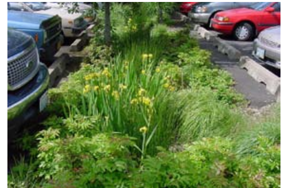
Stormwater Detention Swale
