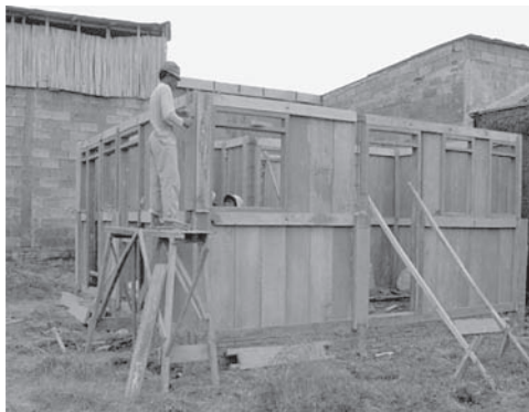
Figure 17. The completion of all prefabricated component assembling.
