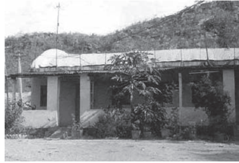
(b) A Finished House with Barrel Roof
