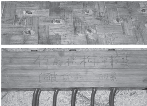
(a) the failure form of main board hole; (b) the flexural failure of bolt.
