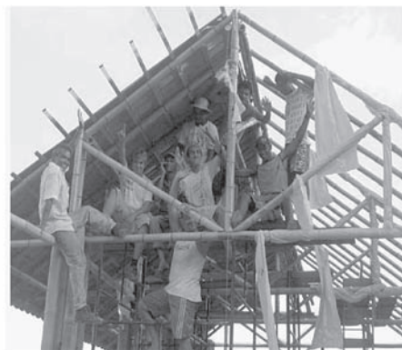
(b) Load testing of bamboo structure
