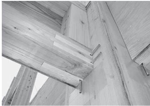
Figure 3. Mechanism of joint using T-type connector.
