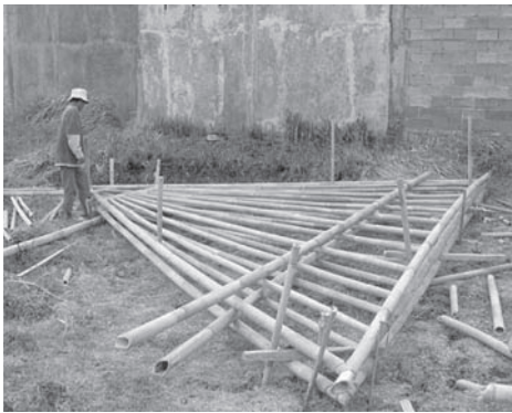
Figure 18. The prefabrication of roof frame on site.
