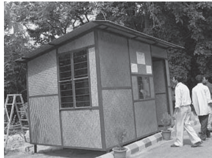
Figure 19. Prefabricated BMB composite house IPIRTI, Bangalore.
