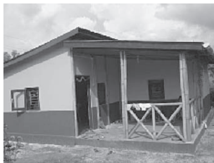
Figure 4. Pre-fabricated bamboo house in Nepal (Courtesy: Himalayan Bamboo).
