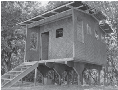
Figure 18. Prefabricated BMB wood shelter IPIRTI, Bangalore.
