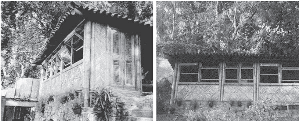
Figure 12. Front and lateral view of bamboo house in Itanhangá/Rio de Janeiro.
