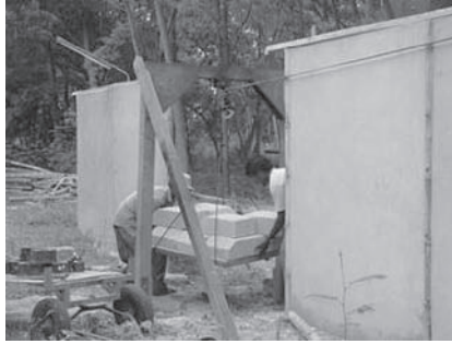
Figure 17. Testing of panels under progress.
