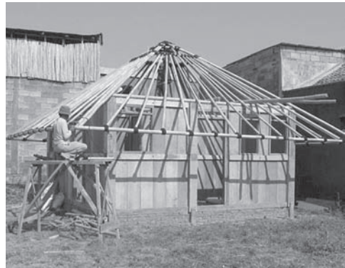
Figure 19. The completion of roof frame assembling.
