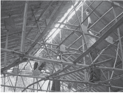
Figure 1. Bow Beam Arches built in 2005.
