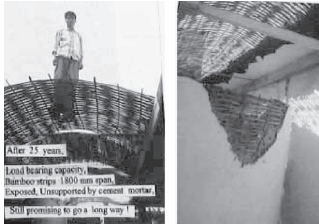
Figure 3. An experimental house with bamboo strips constructed during 1973.
