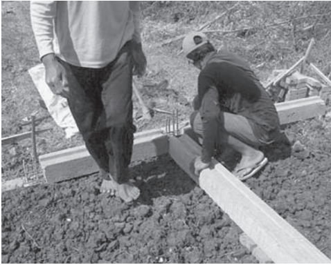
Figure 12. The assembling of prefabricated tie beam.
