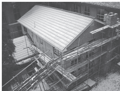
Figure 10. Two-story modern bamboo residential house near completion.
