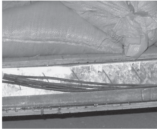
Figure 9. Damage of glue interface.
