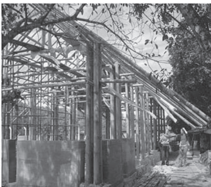
(a) Compacted earth walls and bamboo structure
