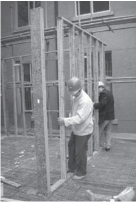
Figure 4. Installation of laminated bamboo walls.
