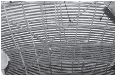
(c) Inside view of the Roof
