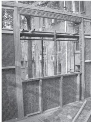
Figure 4. Installation of laminated bamboo walls.
