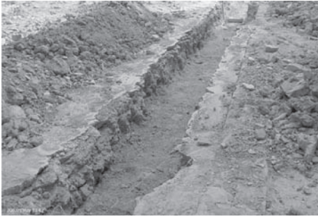
(a) Excavation foundation
