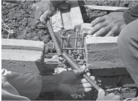
Figure 13. The adjustment of steel reinforcement of tie beam.
