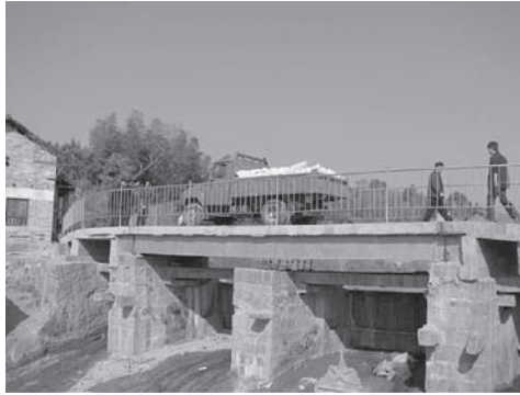
Figure 5. Truck loading test of Leiyang bridge.
