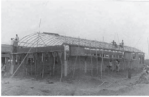
(a) 24 ft Bow Beams for Barrel Roof
