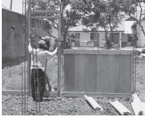
Figure 15. The assembling of prefabricated door frame.
