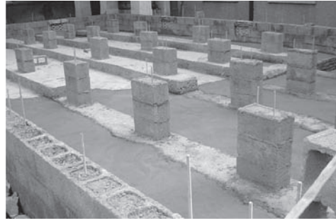
(b) Concrete filled masonry block footings
