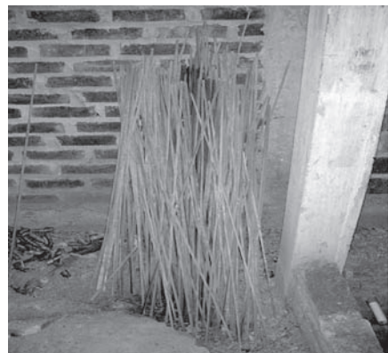
Figure 9. Bamboo splits for reinforcement.
