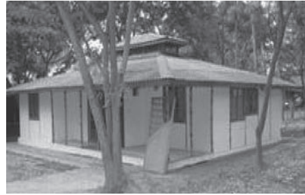
Figure 12. Demonstration two bed room house at IPIRTI—Bangalore, January 2002.
