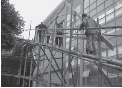
(a) Moving prefabricated truss to site
