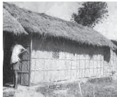
Figure 2. Bamboo house with thatch roof.
