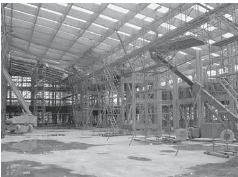
Photo 6. Main hall on construction.
