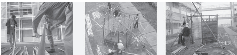
Picture 7. Construction process of shelter 3.
