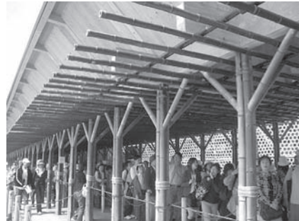
Photo 7. Passage of round bamboo.
