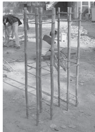
Figure 3. Bamcrete column before casting.
