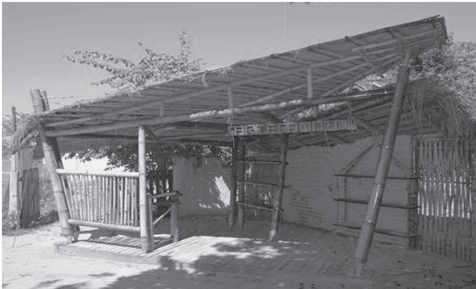
Figure 13. Construction of kiosk using bamboo and earth.
