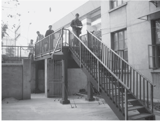
Figure 6. Modern bamboo pedestrian bridge constructed by the authors.
