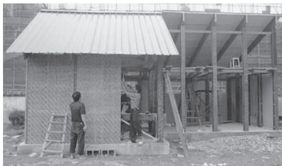
Figure 1. Picture of construction.
