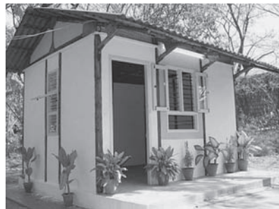
Figure 14. Security House at IPIRTI, Banalore, 2004.
