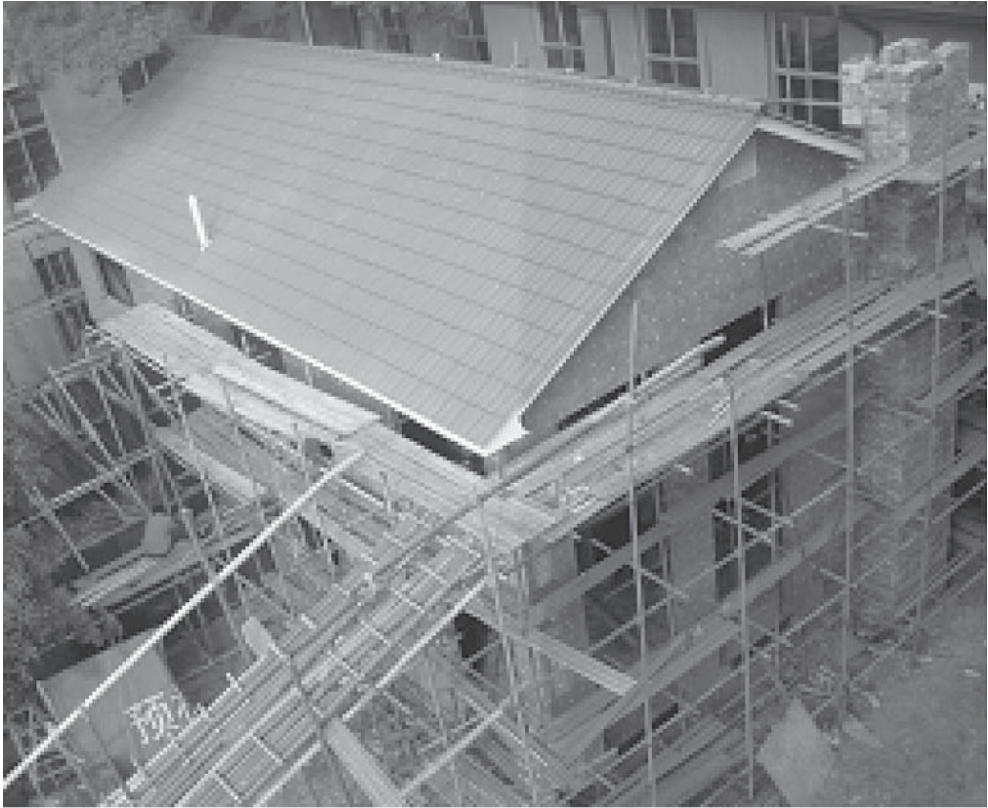
Figure 7. Completion of main structure of bamboo house as of December 2007.
