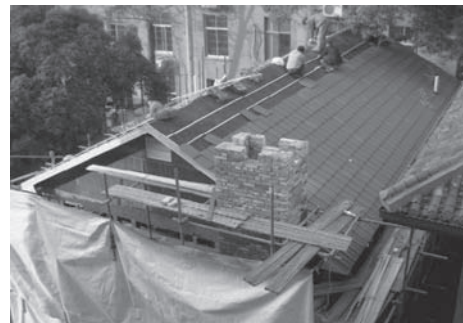
(f) Installation of concrete tiles
