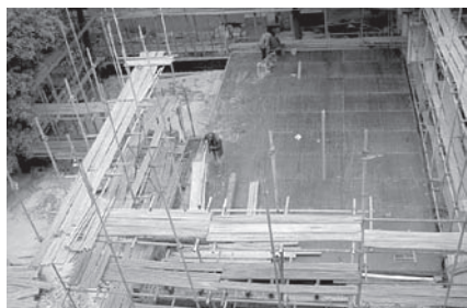
(c) First floor sheathing
