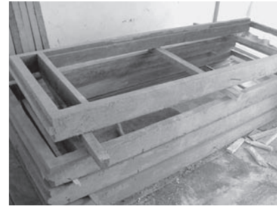
Figure 5. Bamboo RC door frame.
