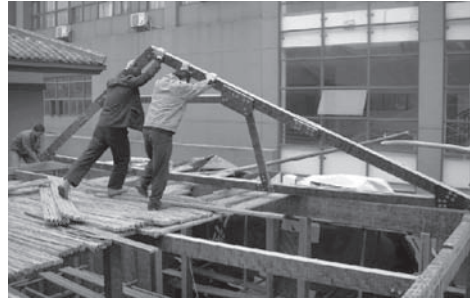
(b) Erection of prefabricated truss
