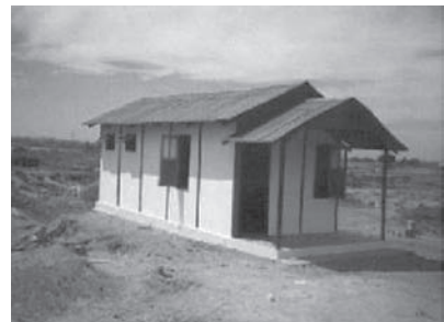
Figure 10. Demonstration House at Chik-kabettahalli, Bangalore, October 1999.
