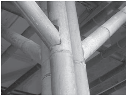
Photo 8. Connection of passage made of round bamboo.
