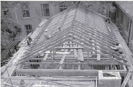
(c) Alignment of roof trusses
