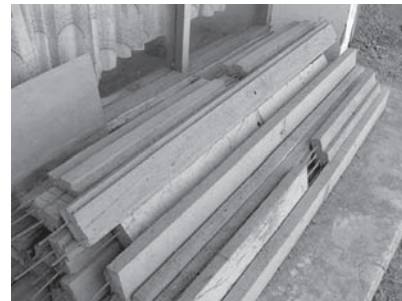
Figure 7. Steel RC middle and top beam.
