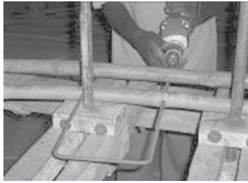
(a) Drilling for the Steel Connector
