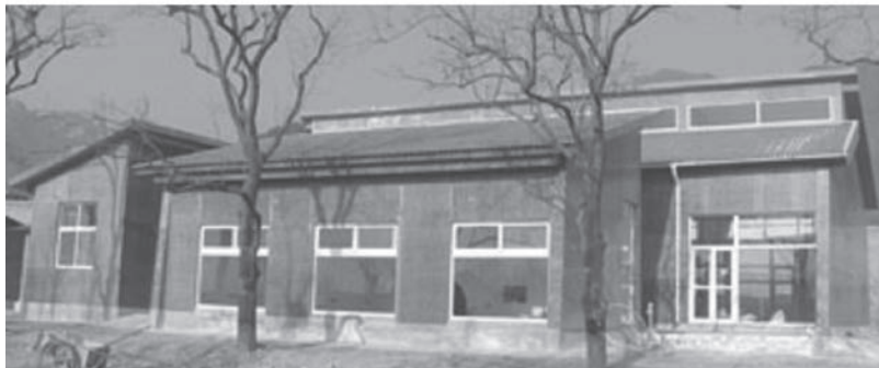
Figure 6. Pre-fabricated bamboo buildings with engineered bamboo (developed and constructed by INBAR) in Beijing.
