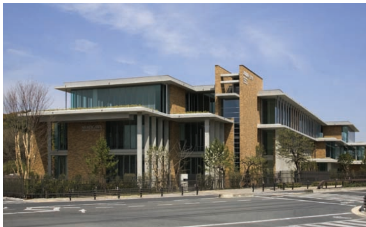
Nikken Sekkei's Architecture Studio at the Architecture Department of Mukogawa Women's University.
