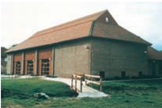
A recently built village hall with an external form and finishes to suit its rural location.
