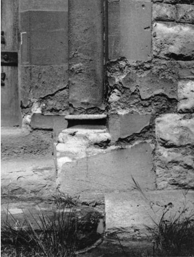
Figure 6.13 Surface blistering of bath stone and Kentish rag stone due to atmospheric pollution.
