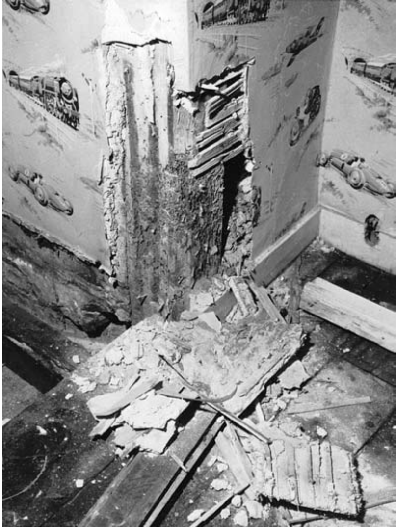
Figure 9.2 Effects of Death Watch beetle (courtesy of SGB Group Publicity).
