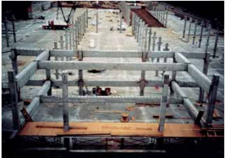
Wide-open spaces can be achieved in parking structures with the hybrid system because it offers lateral load resistance under wind or seismic loads while supplying an open plan free of shear walls.
