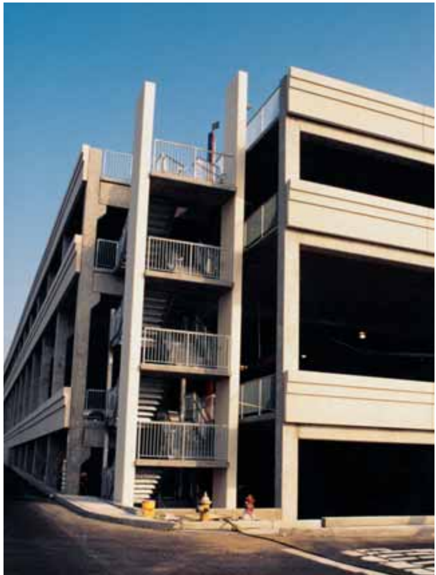
The new hybrid precast moment-resisting frame has been put into practice in a parking structure built at Roosevelt Field Mall in Garden City, N.Y. The system was created in a cooperative effort of Charles Pankow Builders Ltd., the University of Washington, and the National Institute of Standards & Technology (NIST).
