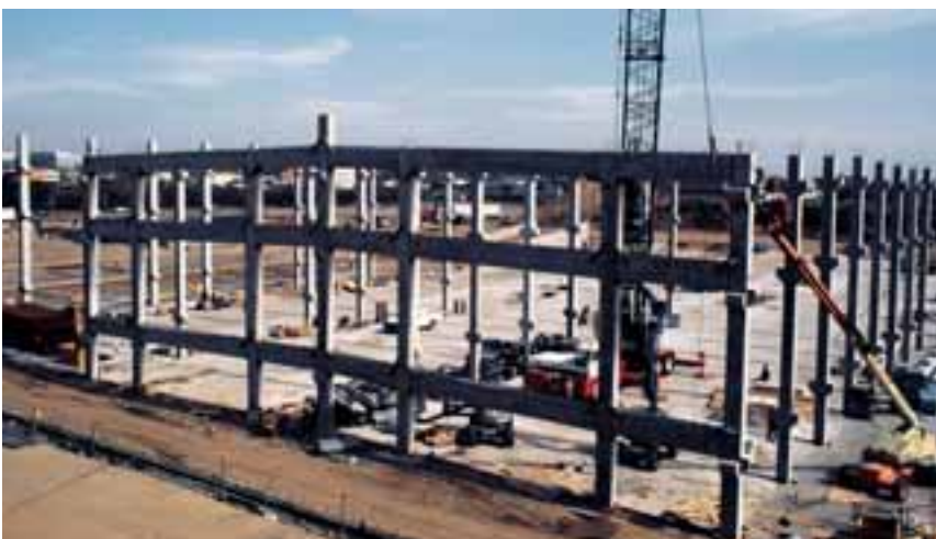
The connection system opens new possibilities to designers because it will make precast concrete construction in high-seismic zones faster and more economical.
