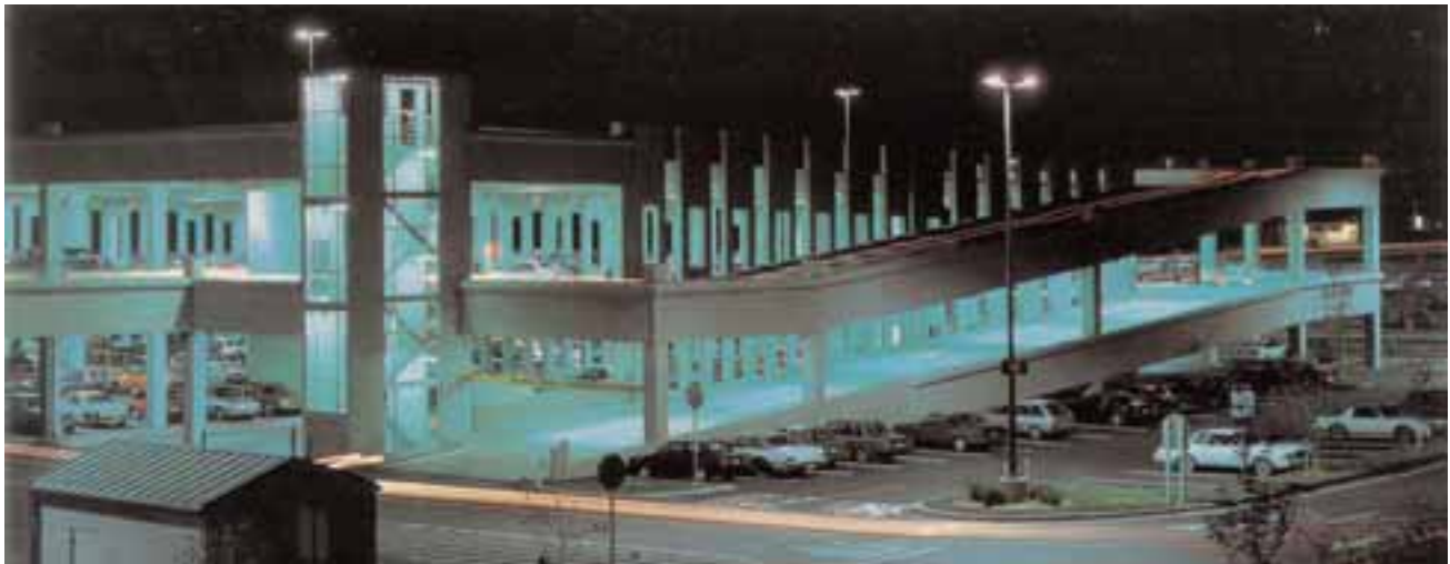
Emerald Mall Parking Garage.
