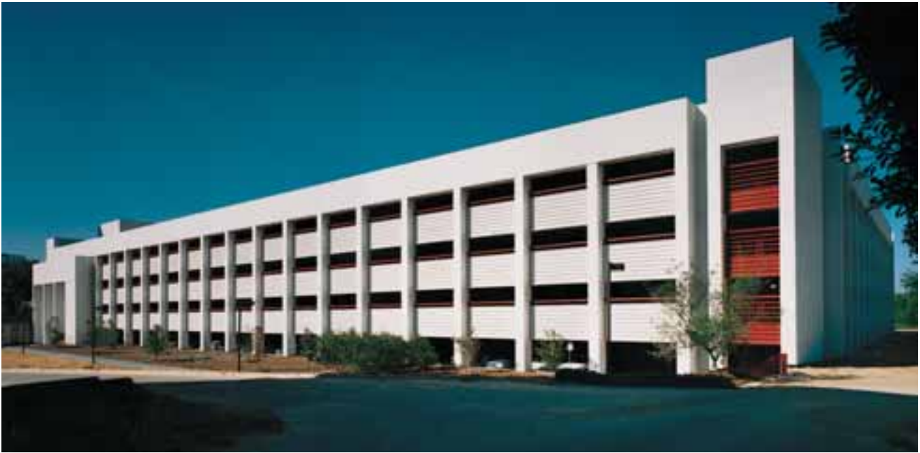
Primary design consideration focused on the deck serving as the background for present and future building sites. Photo: Joann Sieburg Baker
