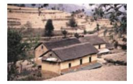
Passive solar orientation and shading maximises solar gain. East and West glazing is omitted. Walls of rock collected from farm terraces are high in thermal mass and blend with the landscape (they are annually rendered with mud in colours of the landscape). This guarantees longevity and prevents heat loss by caulking cracks and crevices. Early Australian settlers used similar building methods. [See: Passive Solar Heating]
