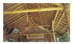
Indonesian vernacular buildings use thatch as high level insulation to deal with heat gain in a tropical climate. Open gables allow cross ventilation of the hottest air that would otherwise accumulate in the roof space. Generous eave overhangs shade the building, further reducing heat gain. These principles are employed in the traditional "Queenslander" which is also an excellent example of climate responsive architecture.
