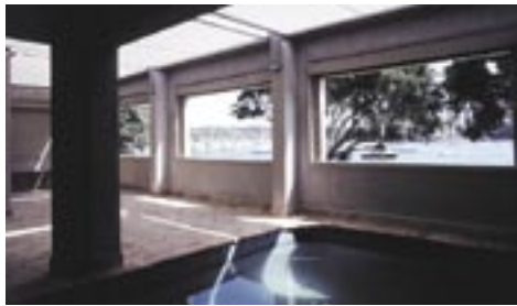
Air enters this building across the pool (thermal mass) via a semi-enclosed courtyard. It is evaporatively cooled before entering the building
