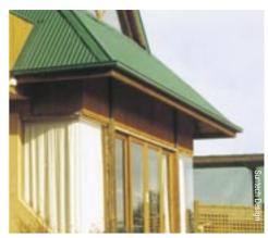
Above, standard 2100 high doors are shaded by a 1000 eave (including gutter) set 300 above the head. Note the sun angle at midday in mid winter is above the glass line. This configuration provides full shading to glass from late October to late February at latitude 35°S (near Canberra) and is appropriate for a higher altitude cool climate winter.
