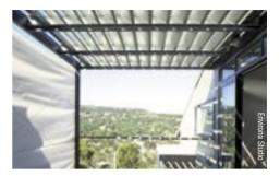
Adjustable shading appropriate for northern elevations includes adjustable awnings or horizontal louvre systems above glazing, and removable shadecloth over pergolas or sails. Shadecloth is a particularly flexible and low cost solution.
