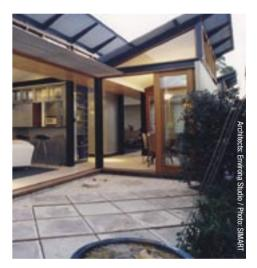
Above, north facing upward raked eaves allow full exposure of glass to winter sun and shade larger areas in summer, without compromising the solar access of neighbours to the south. This inner city terrace in Sydney uses an upward raked eave to passively shade highlight windows. A separate horizontal projection of louvres shades lower glazing. This allows 100 percent winter solar access and excludes all sun between the spring and autumn equinoxes.
