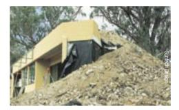
Earth covered: High embodied energy; high thermal mass with excellent thermal performance from earth-coupling, no insulation required in many regions (dependent on soil temperature at various depths). Capable of zero heating and cooling energy; maintenance free; very durable when waterproofed correctly; high site disturbance during construction, minimal on completion. High cost.
