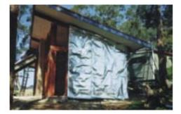
Reverse masonry veneer: High embodied energy with clay bricks, low to medium with concrete block. High thermal mass and high thermal performance with added insulation. Low internal maintenance, external maintenance dependent on finish. Very durable and re-use potential fair. Range of environmentally preferred external cladding includes fibre cement, plywood, sustainably sourced timber or colourbond steel. Cost varies with mass type, which can be any masonry.
