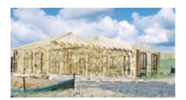
Brick veneer is an inefficient, high embodied energy cladding system. The brick has no structural role. The above photograph shows a lightweight timber framed home structurally complete and ready for brick cladding. If this home was clad with lightweight, low embodied energy materials, its structural and thermal performance would be unaltered. Its embodied energy would be lowered along with its cost. [See: Thermal Mass]
