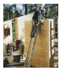
Rammed Earth: low -medium embodied energy, depending on cement content. High thermal mass; poor insulation (difficult to add unless lined externally as above); minimal transport energy when used on remote sites, minimal manufacturing process impact, very durable but requires some maintenance (reapplication of waterproofing), average to high site impact, depending on footing system. High cost. [See: Construction Systems - Rammed Earth (Pisé)]
