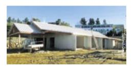
Sandwich panels have varying embodied energy depending on surface materials and insulation. Those in the photograph above are fibre cement outer linings with EPS studs and concrete core fill. The concrete fill adds thermal mass and an outer layer of insulation yields excellent all round thermal performance.
