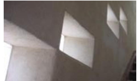
This dry-lined interior shows how AAC can be exploited to make niches and unusual openings.
