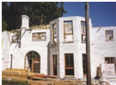
Block construction showing two storey house
