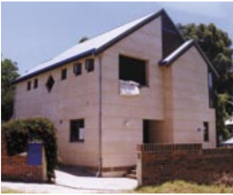
This Perth home is one of Western Australia's many fine examples. Rammed earth has a long life expectancy and is ideal for buildings that are intended to survive for many decades.
