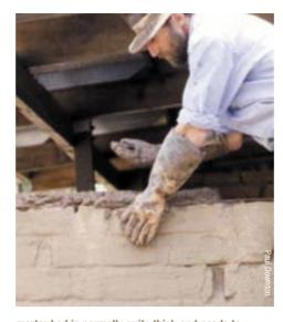
mortar bed is normally quite thick and needs to provide complete bedding for the bricks. Perpends are similarly thick (about 20 - 30mm). The intention is to produce a wall that is effectively monolithic, ie. as if it were a single piece of material.
