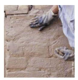
After brushing to get a fairly even surface, the final finish is a mud slurry, typically finished by hand. This slurry may also be the final waterproofing coat (eg. A mud and cow dung mix) or it may have a further clear coat of proprietary waterproofing material. Linseed oil and turpentine can be used to provide a final finish.
