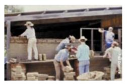
The clay content of adobe can range between 30 and 70 per cent and the overall earth content may also include silt, gravel and stones. There are a number of tests for suitability of the earth and the approval process may require an erosion test. Before excavating for on-site mud, consider the site layout to minimise carrying and transport and ensure there is space to keep any topsoil separate for use on the garden.
