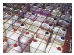
These void formers are mostly expanded foam boxes, which interfere with earth coupling, but more thermally connective alternatives are available. These include proprietary systems that use recycled tyres, or reused detergent bottles filled with water and grouped together as void formers.
