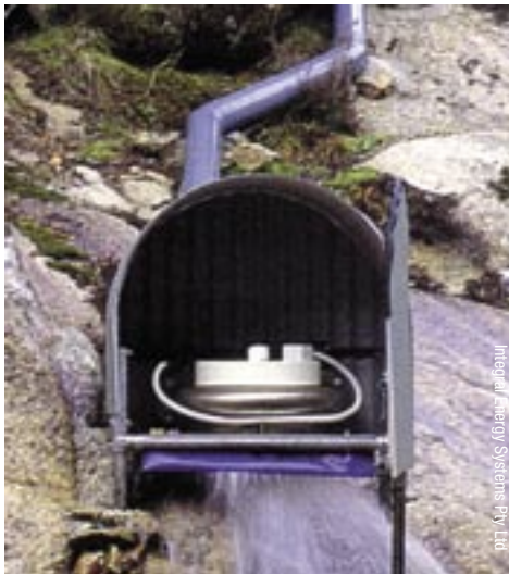
Typical micro hydro system.
