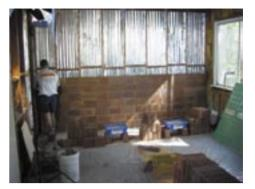
Almost any bricks are suitable for RBV construction, but Austral 90mm SlickBricks were selected for this project because of their slender width, which consumed less floor space. Second-hand bricks are ideal if available.
