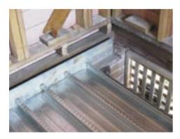
This type of slab uses the existing piers and footings, and requires no filling or excavation. The concrete is poured over prefabricated steel decking. The slab was installed lower than the original floor to gain extra ceiling height.
