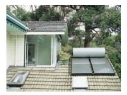
The hybrid system comprises an un-boosted 300 litre Edwards Stainless solar heater and a high efficiency 130 litre Rheem Stellar gas storage heater. [See: Hot Water Service]
