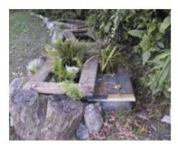
The waste water is fed up through this matrix, overflowing at one end into the bottom of the next tank, where the same process is repeated, and again into the third tank.
