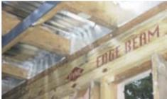
Engineered timber allows these longer spans to be handled with minimal member depth. A laminated 200 x 45 mm timber beam called a Hyne Edgebeam LGL was used in this instance.
