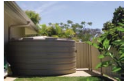
The 5 kL rainwater tank
