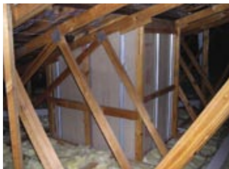
Roof framing: plantation softwood. Note the skylight shaft to the family room
