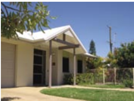
Entrance, facing N/W, well shaded
