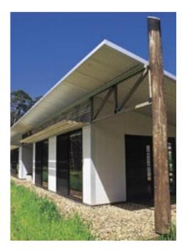
The roof panels are made from "Ritek", a sandwich panel of two corrugated zinc alum steel sheets bonded either side of a 100 mm thick sheet of EPS foam. The truss to the north side is clad on both sides with clear polycarbonate sheet, allowing the structure to be seen from inside and outside but providing passive solar gain through a virtual double glazed panel.
