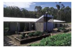
Modular components were used in the design, fabricated offsite to minimise waste and to allow simple, speedy erection of the house. A 1200 mm modular grid is used throughout to standardise material sizes based on commonly available sheet materials and windows and doors. Sculptures at either end of the long walkway emphasise this eastwest axis whilst internal covered courtyards provide visual axes in the north-south direction opposite the bathrooms. [See: Construction Systems, Waste Minimisation]
