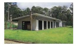
The outdoor area to the north of the house is maintained as a gently sloping grass area that allows for maximum solar access and provides bushfire protection. To the south, the house has been dug slightly into the hill providing protected courtyards that received winter sun but are protected by the embankments and planting to the south.
