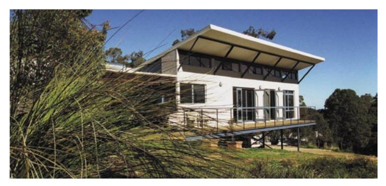
expensive partially elevated concrete slab over a full slab on ground to achieve this. This construction also allowed for the house to be on a single level.
