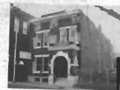
Ely Building Knoxville, TN
